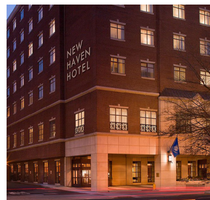
New Haven Hotel New Haven, CT
